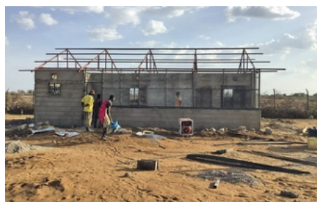
The second mission building is under construction
