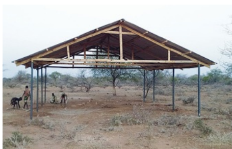
School building under construction
