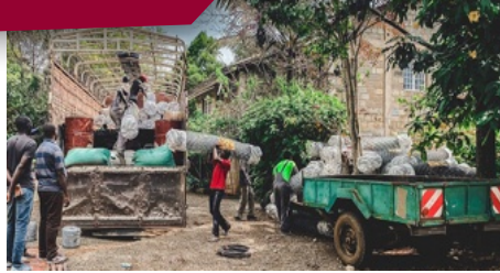
The construction of the base in South Sudan is progressing! 4
