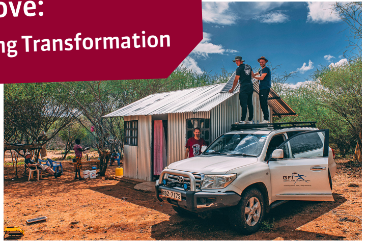
Installing a solar panel on Mary's roof
