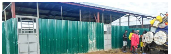
Fertige Halle in Loitmor/Sudan
